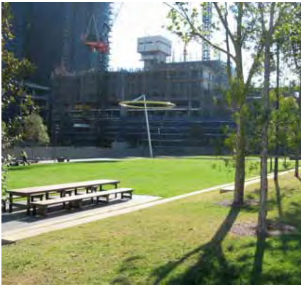
< Construction underway at CUB site.
